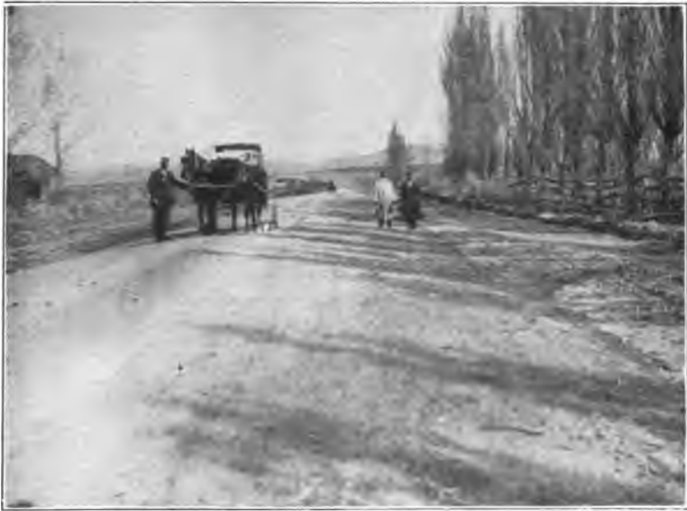
FIG. 8. ROAD SCENE LOOKING NORTH TOWARD MORONI, SHOWING THE ADVANTAGE OF USING ONLY A PORTION OF THE STREET FOR ROADWAY
